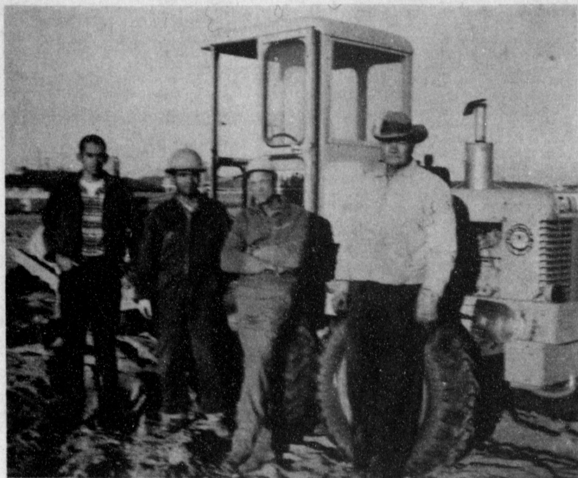
BUILDING COURT --City employees began the ground work this week on the plot where the tennis courts are to be, south of Municipal Swimming Pool at the High School. Shown here are four of the workmen, Duane Ham, Roy Torres, L. M. Bell and Ernest Martin. They are hauling sand in and leveling it with the maintainer.
