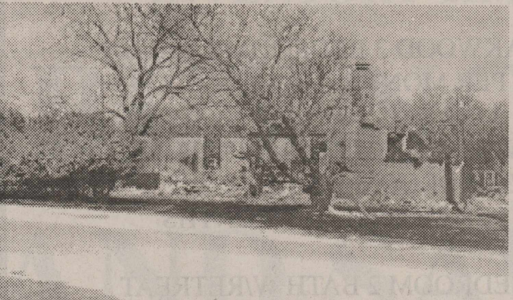
LARGE BRICK HOME — in north Cross Plains destroyed by flames.
