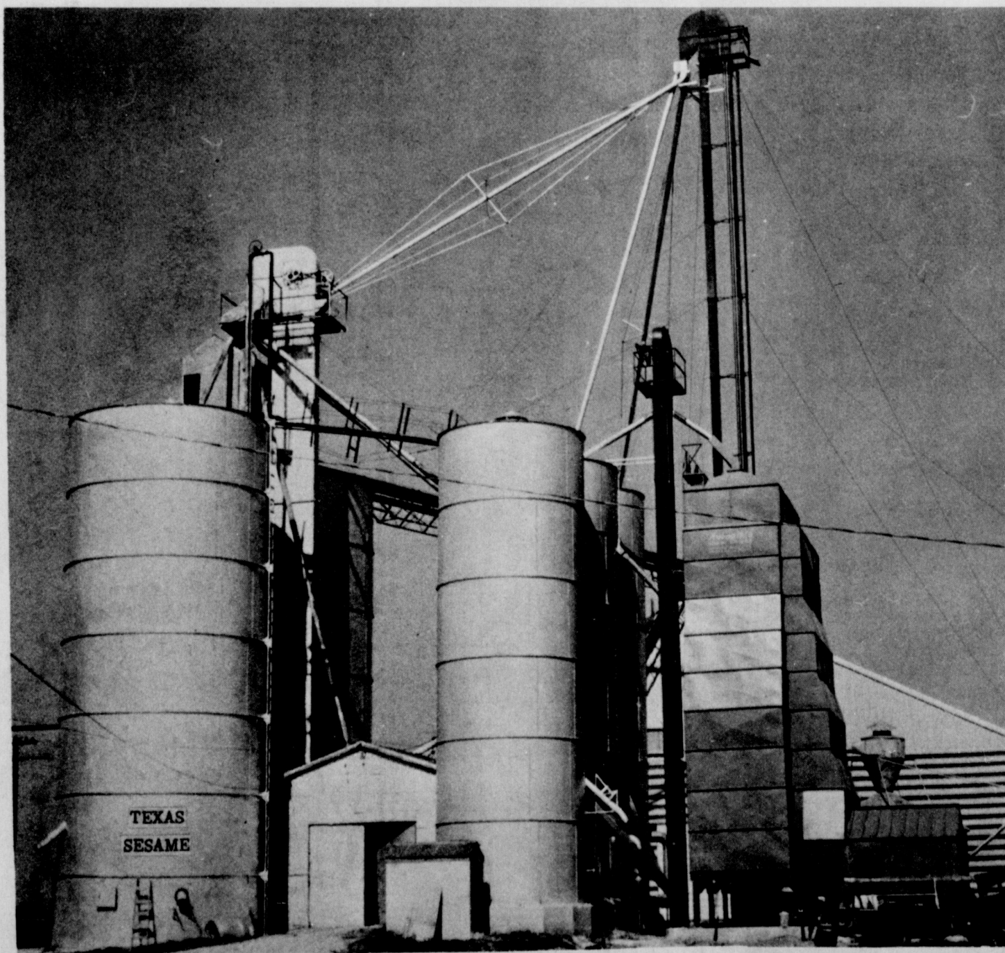
PROGRESS INSTALLATION Largest Corn Dryer South of Kansas City.
