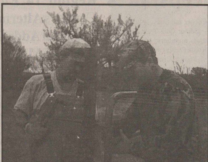
WORKING HARD —Phillip Bennett (left) and Bryan Bennett (right) made repairs to one of the cemetery gates.
