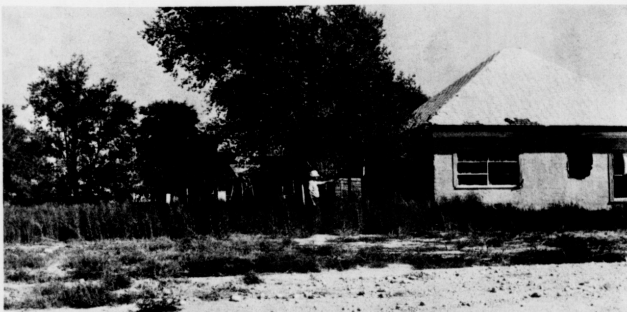
FIRE HAZARD--Here Fire Marshal Owen Jones points out a vacant house with windows knocked out and surrounded by weeds.
