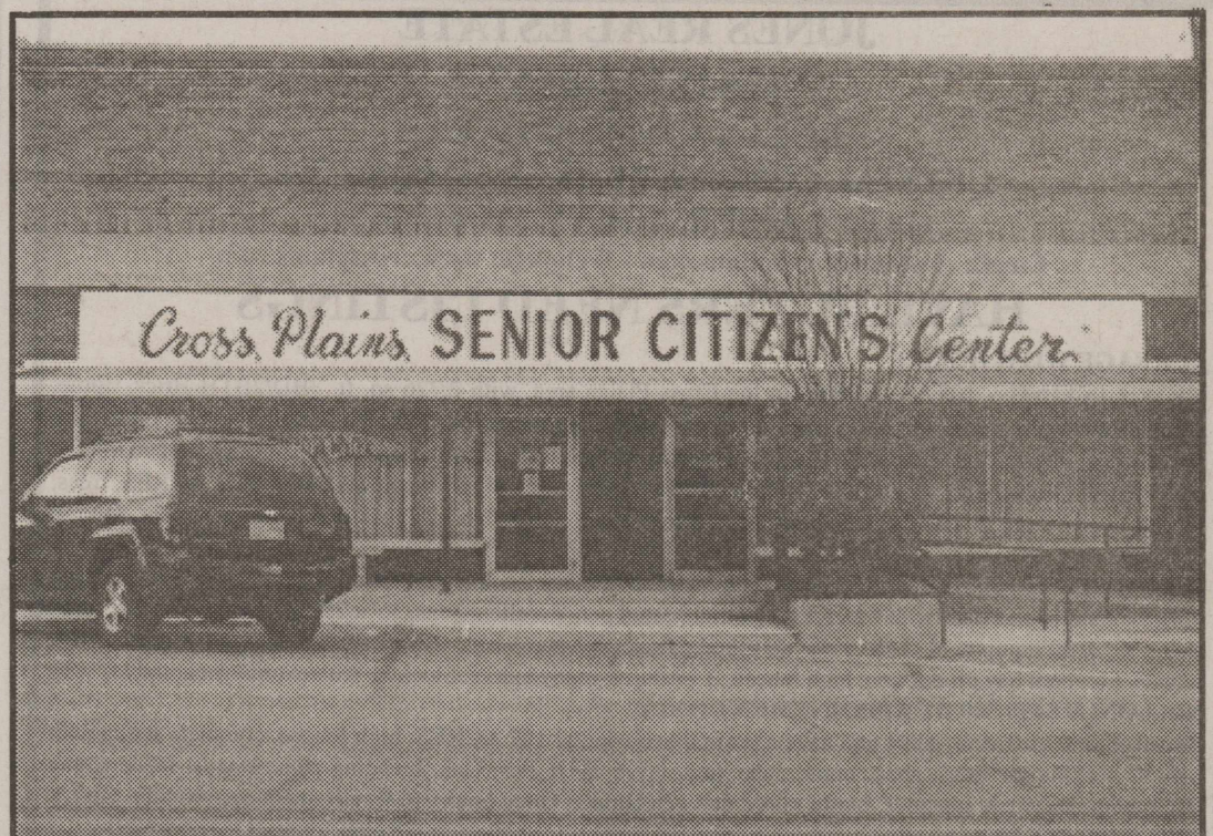
LOOKING GOOD— The Cross Plains Senior Citizen's Center has a newly painted sign and metal awning on the front. The Cross Plains EDC contributed $750 toward the project and the Senior Citizens of Cross Plains Renovation Fund Committee picked up the balance. Davy Crockett donated his time to repaint the sign, while the Committee furnished the paint. Rex Beggs and his son-in-law Gary Moses built the awnings.
