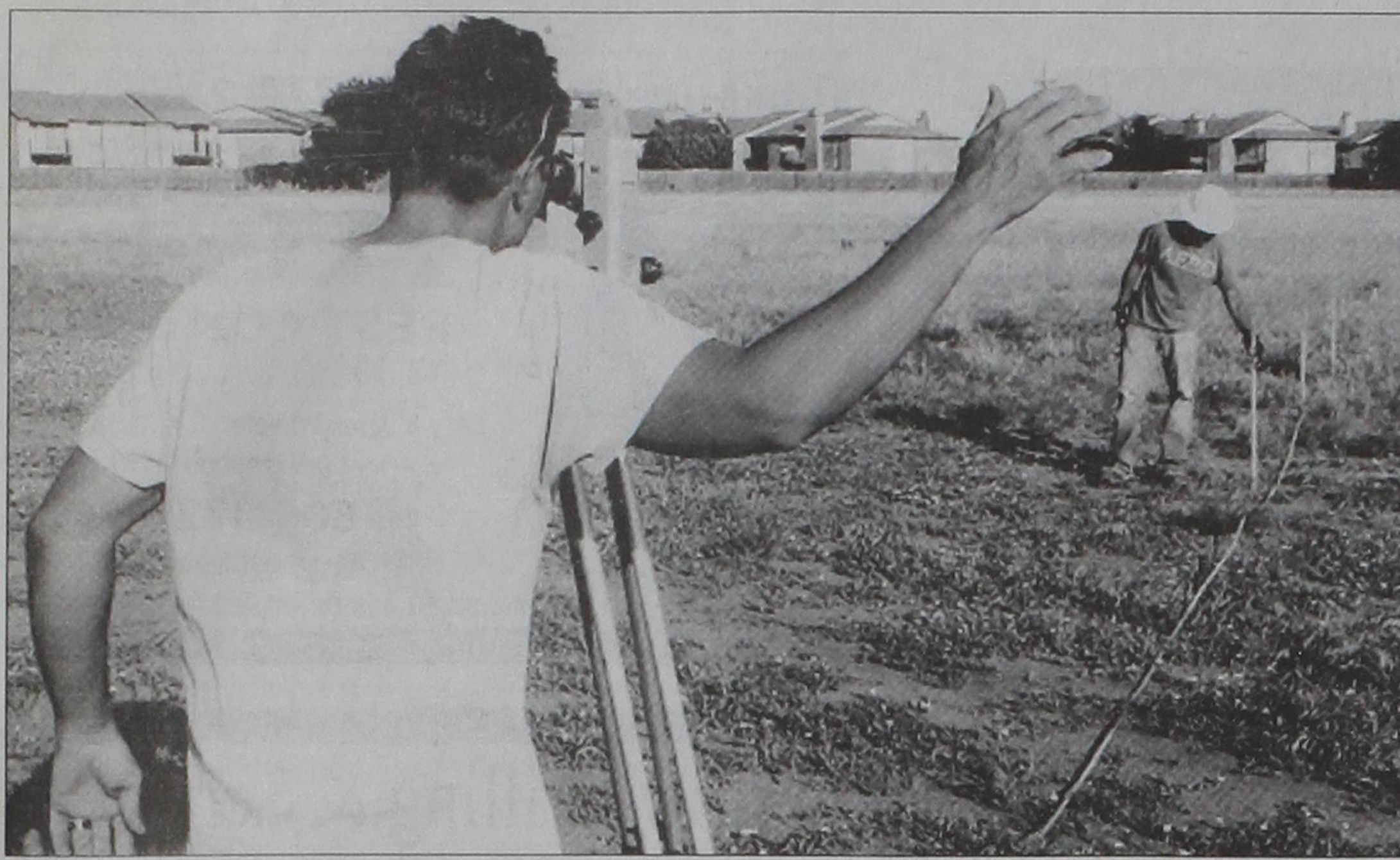
Micah Nichols and Jerome Wheeler, of Cielo Wind Power, LP, survey and stake the location at Clarendon College Pampa Center where a 50 foot MET tower will be erected.
