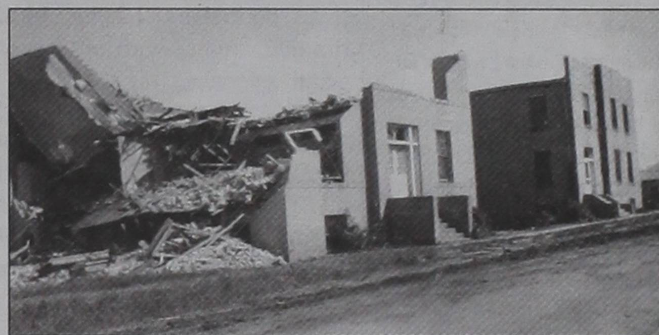
Looking at the west side of the Girls Dormitory, provides a closer view of the damage. Building caretaker Tom Tucker received a deep gash in his head from flying glass but counted himself and his family lucky.
