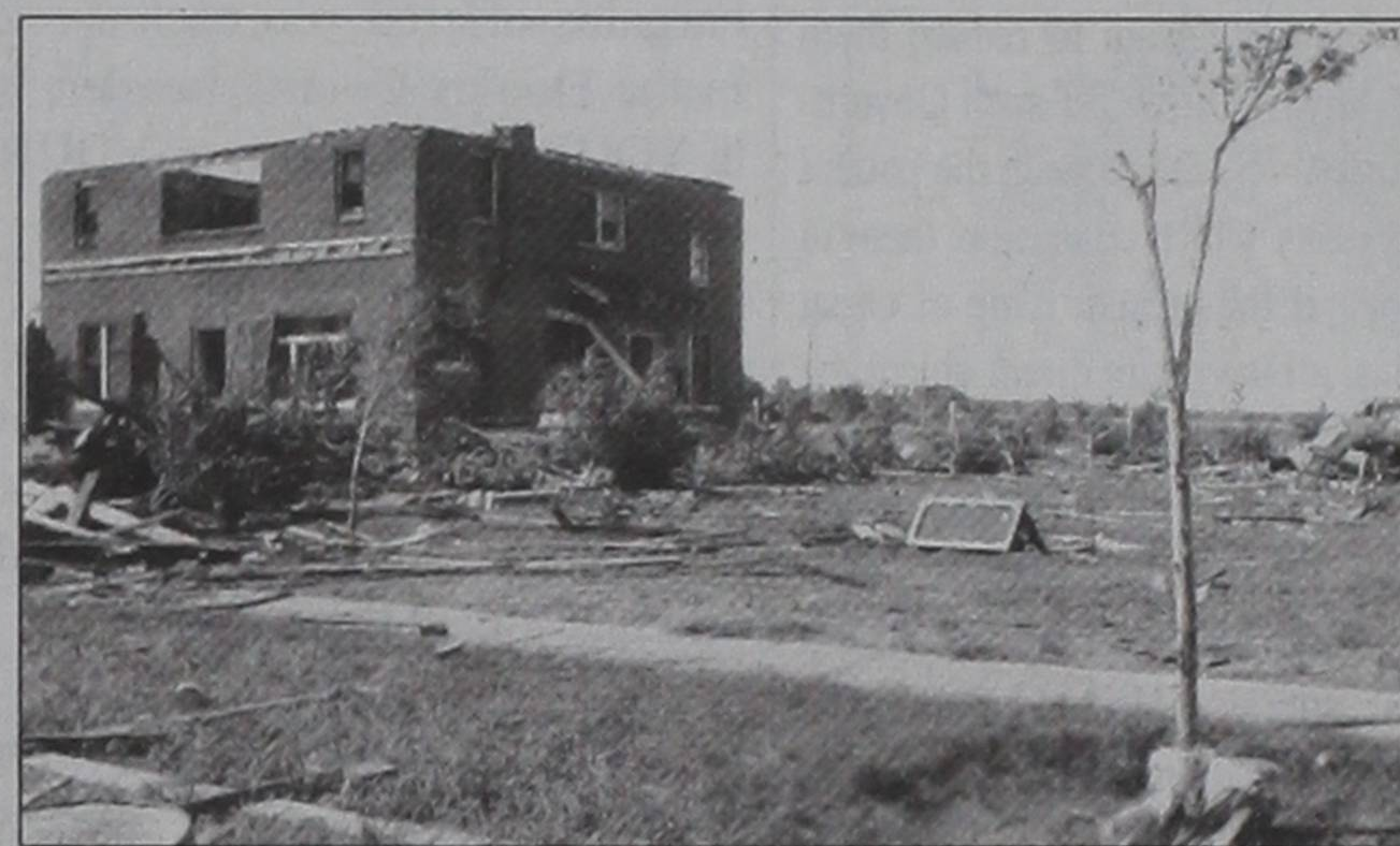
The home of Mrs. Lena Antrobus (the current home of Terri Floyd) was a ruined shell after the tornado. Before striking this home, the storm blew down the east wall of Broncho stadium, an almost completed $30,000 WPA project.
