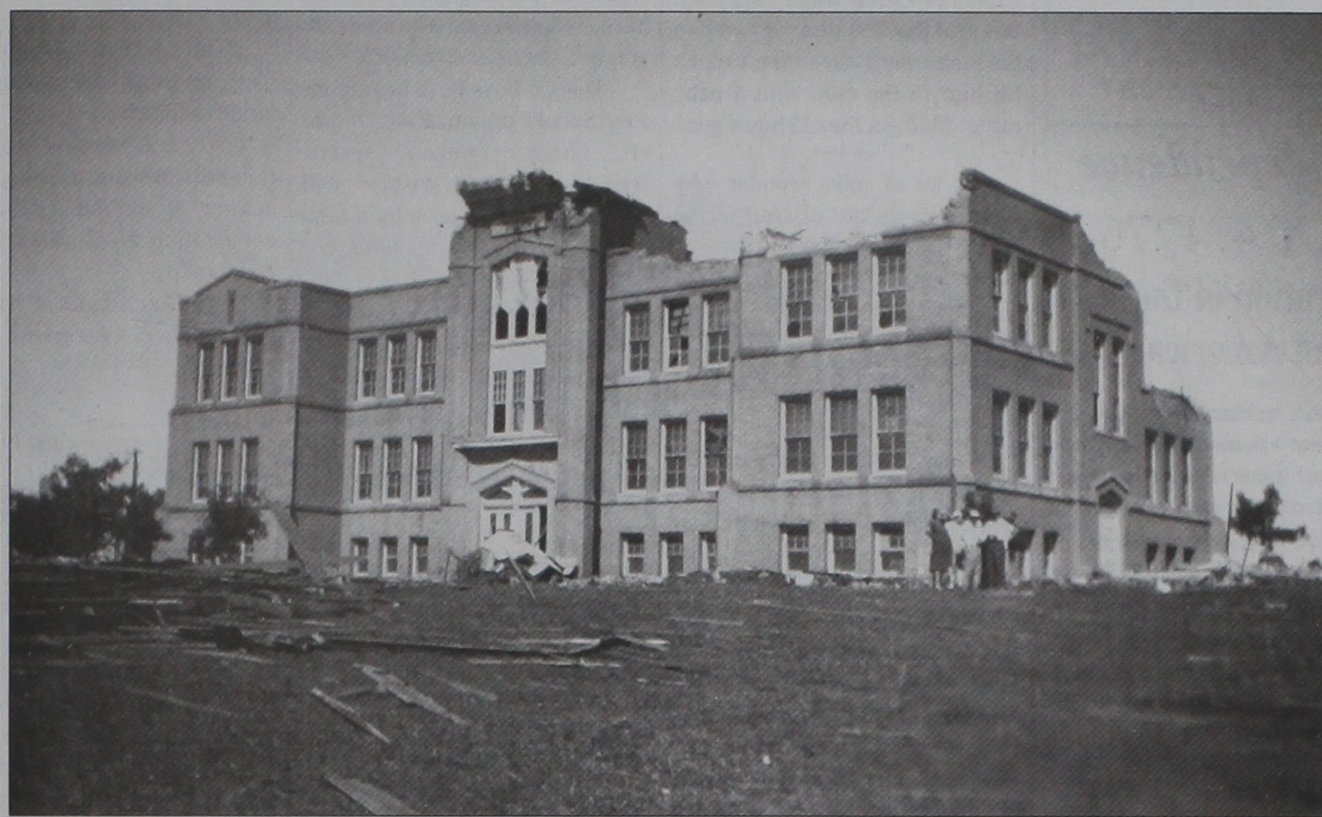
SHATTERED RUINS Mark Disaster's Path - Monday, June 9, 1941 - The Panhandle's oldest institution of higher learning, Clarendon College, was hard hit by the tornado blast. Destruction to the main building was much more severe than can be seen in the picture above.
