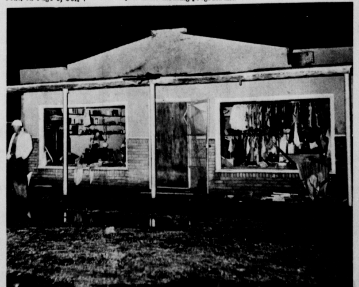
TORNADO!--At 8:11 Tuesday evening, a tornado dipped down at the south edge of Earth and among the damaged buildings and homes was this TV Repair Shop. Also receiving damage were a warehouse, an implement company, several homes and barns. No injuries were found from the tornado, however, one woman was hospitalized following a heart attack. Law enforcement officials, civil defense workers and fire department personnel from many areas converged on the community to assist.
