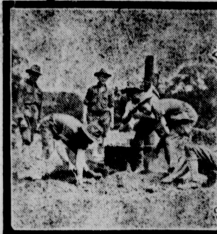
Digging a Trench for Drainage is Necessary in the Sanitation of an Army Camp.
