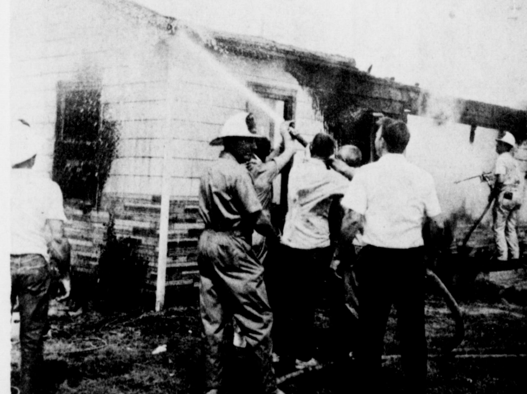
FIREMEN BATTLE BLAZE--Members of the Bailey County Volunteer Fire Department wage a futile battle in an effort to combat a blaze which destroyed the home of Rev. Arthur Hayes Sunday afternoon. The fire went undetected until it had broken through the roof of the home. Fire Chief Earl Ladd said the fire started in the kitchen area due to unknown causes. The family of four lost everything they owned except the clothing they were wearing.
