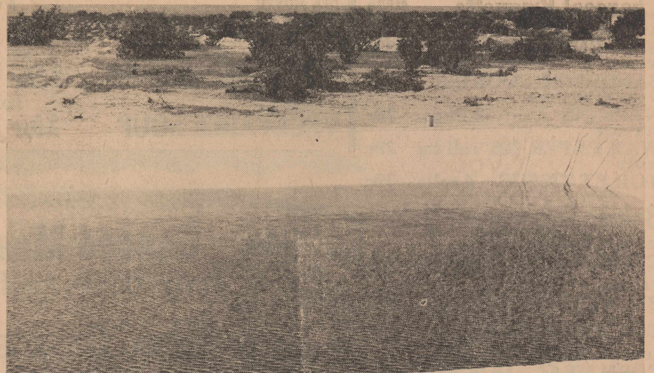
THIS VINYL LINED pond collects the plant waste waters, largely cooling tower blowdown of about 2200 parts per million total dissolved solids, for injection underground to prevent shallow fresh water pollution.
