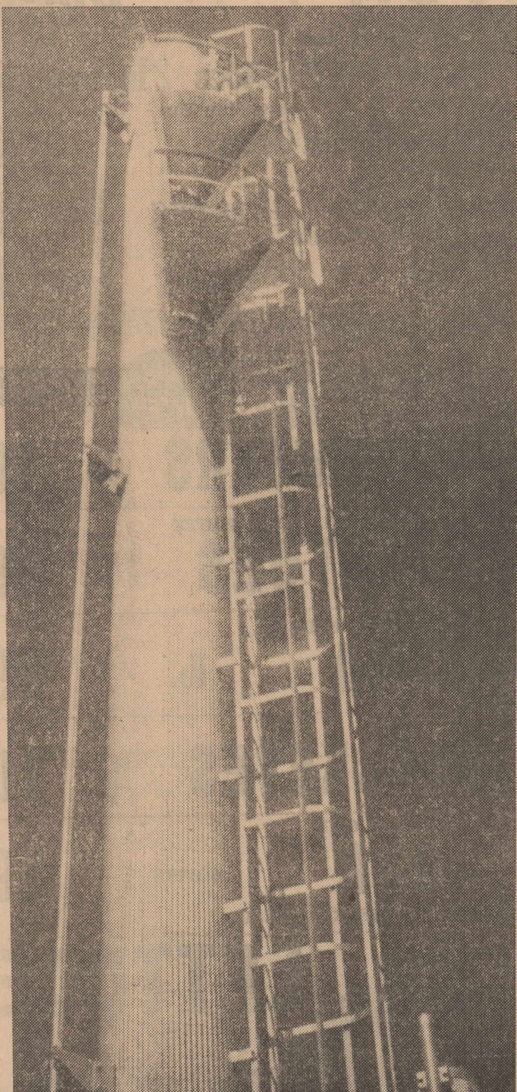
UP, UP, UP the deethanizer and debutanizer columns rise above the area. In these columns the feed is fractionated into LPG and natural gasoline products.
