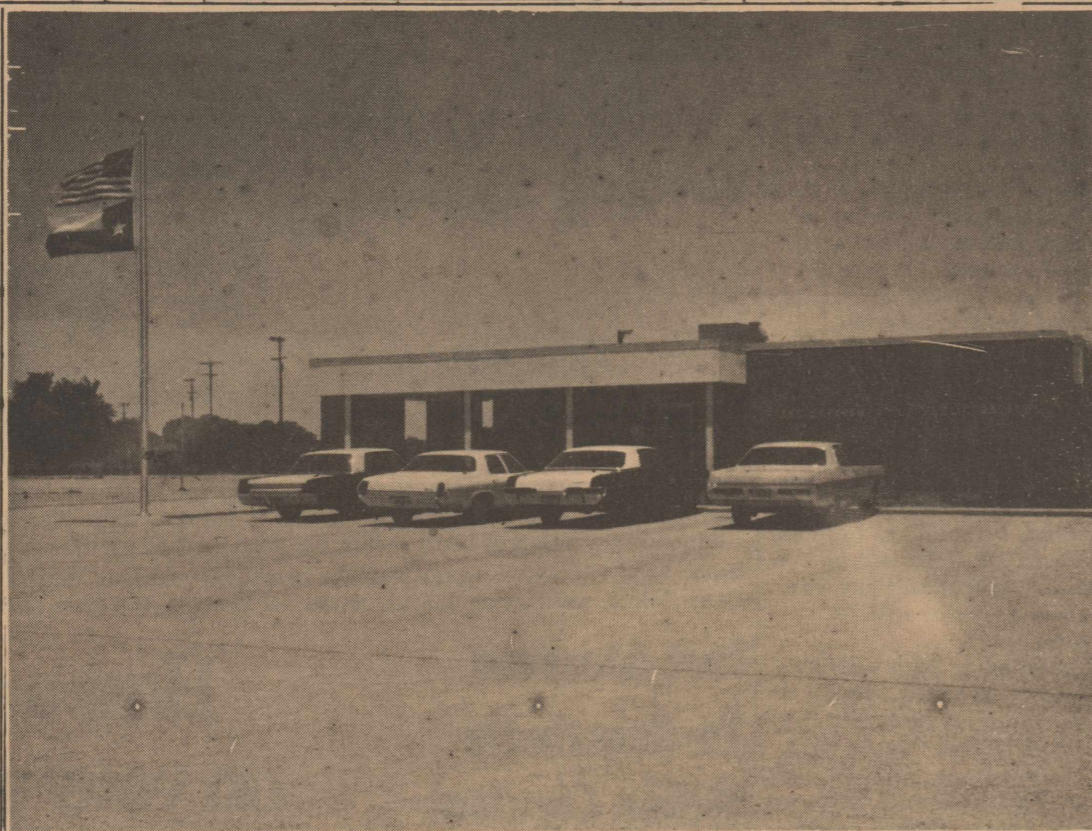
DPS COMMUNICATIONS CENTER in Ozona was dedicated Friday afternoon by Colonel Wilson E. Spier, director of the Department of Public Safety in Austin. Col. Spier said the strategically located local facility will contribute much toward better law enforcement in the state.
