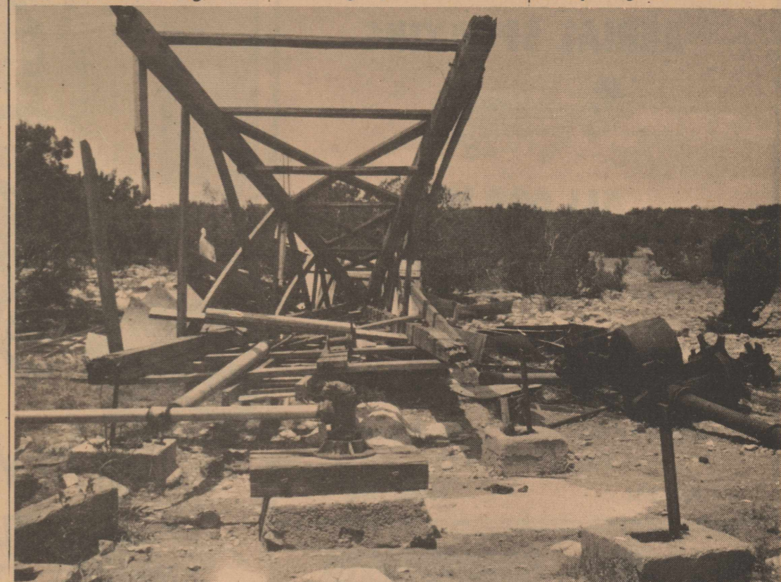
HIGH WINDS demolished this windmill on the Joe Couch ranch Thursday night before a brief rain shower. The freak wind snapped the wooden structure off at the base, along with connecting pipes and smashed the whole thing to the ground right next to the foundation where it originally stood.
