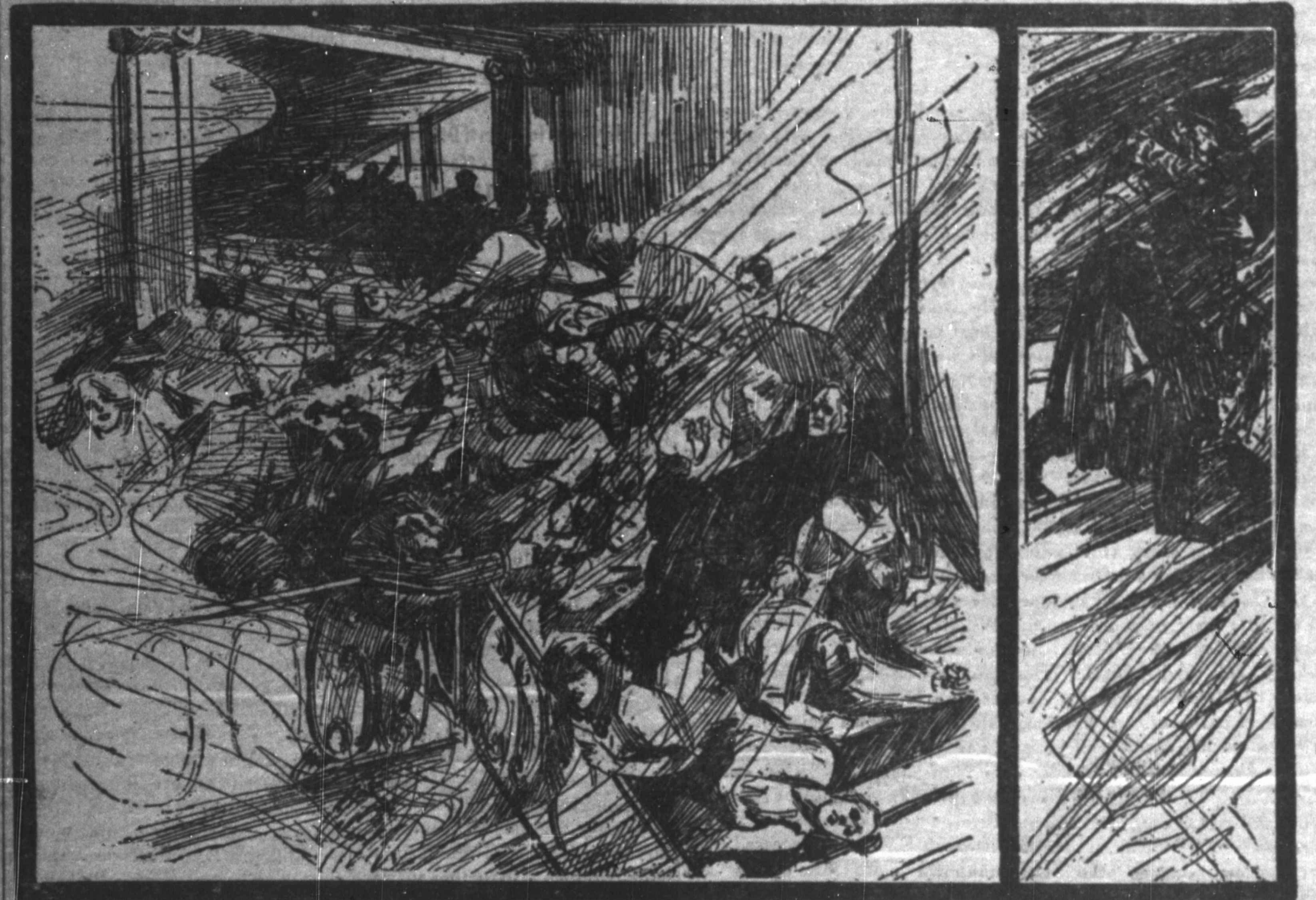
Death Trap at Main Balcony Exit.
