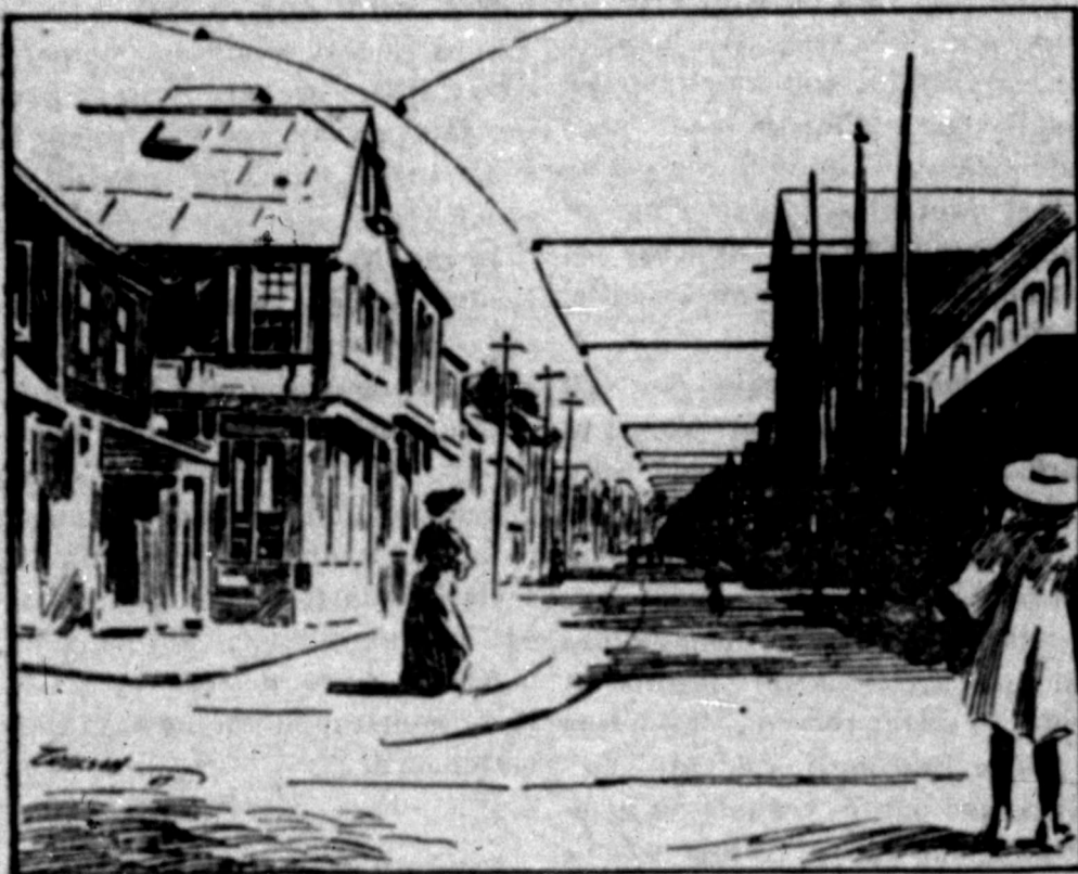
East Street, Looking Toward the Water Front. This Section Was Completely Devastated by the Earthquake and Fire.
