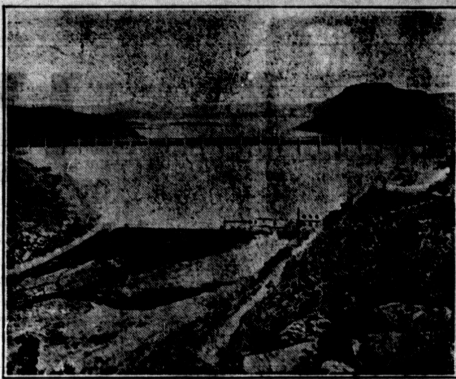
ELEPHANT BUTTE DAM, NEAR EL PASO, TEXAS. 1310 FEET LONG AT TOP, 16-FOOT DRIVEWAY. LARGEST CONCRETE, GRAVITY TYPE, DAM IN WORLD. CAPACITY 115,098,000,000 CUBIC FEET OF WATER—LARGEST ARTIFICIAL LAKE IN THE WORLD—WOULD COVER DELAWARE WITH WATER TWO FEET DEEP.
