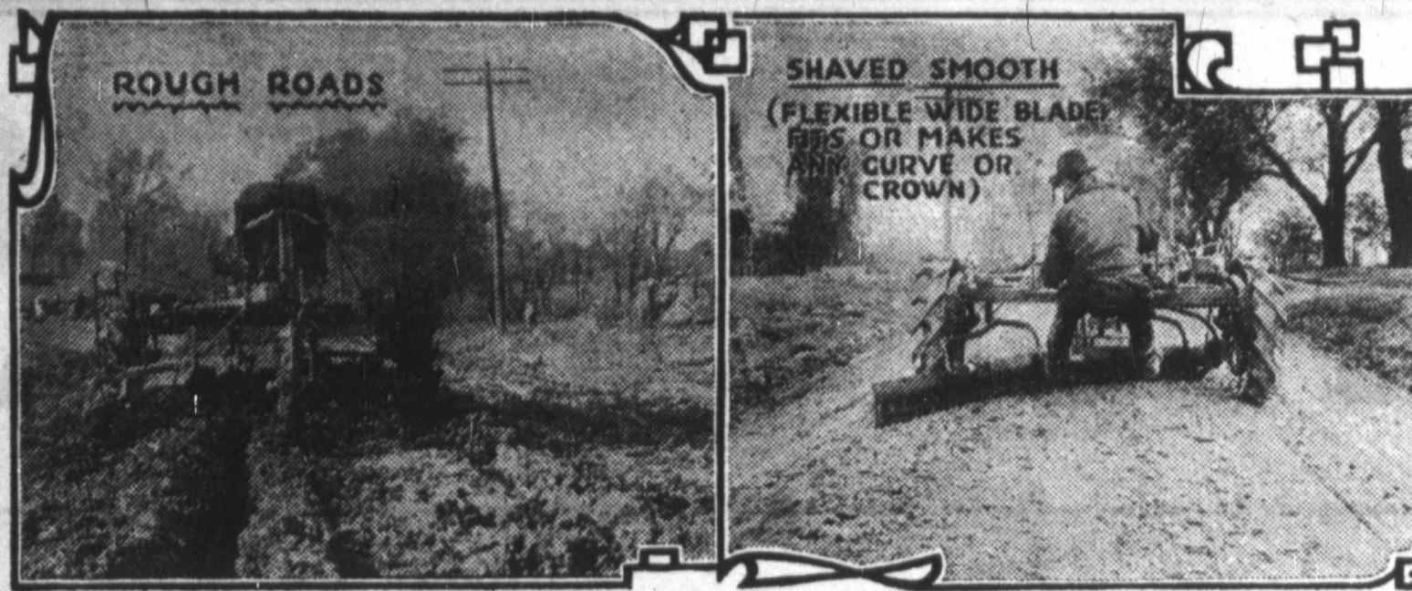
ROADS BEFORE AND AFTER SCRAPING.
