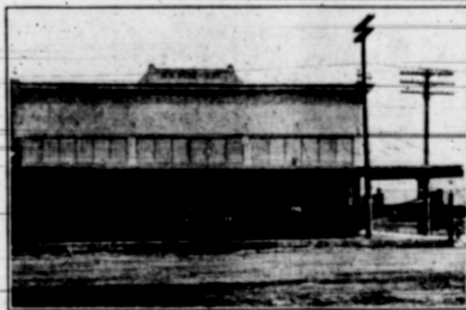
Store of D. G. Vick. Two Plate Glass Windows Were Broken Out in the Storm.
