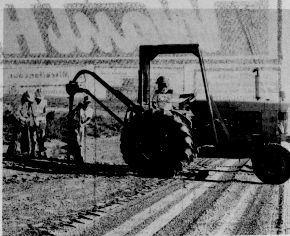
DIGGING NEW FENCE HOLES...On the tractor, Becky Via of Abernathy prepares to lower the digger for new post holes where a fence is under construction on the back side of the Muleshoe National Wildlife Refuge. She is a work leader for the 20 youths at the refuge. Also pictured are Judy Morgan, Three Way, Pam Kirk, Amherst and Gloria Simpson, Three Way.
