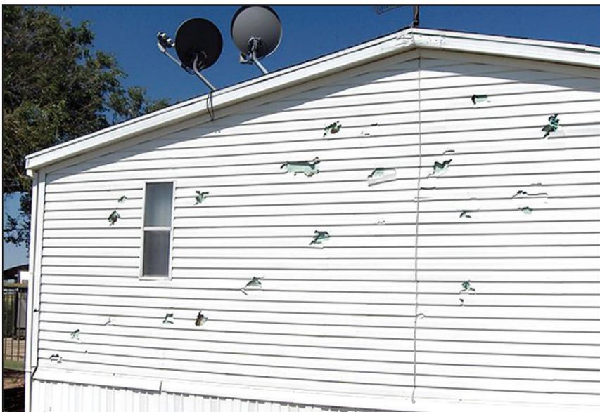
Pictured above is the east side of the Foley residence. Pictured to the left and below is the interior wall damage, and below that is one of the large hail stones that caused the damage.
