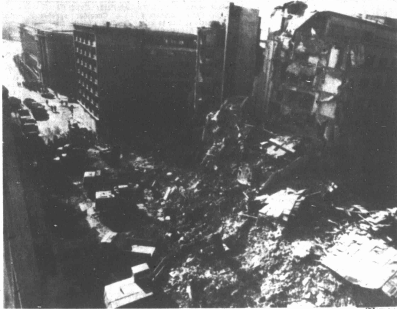
Main streets of Bucharest are blocked by debris from apartment and office buildings in the aftermath of the massive earthquake Friday night.
