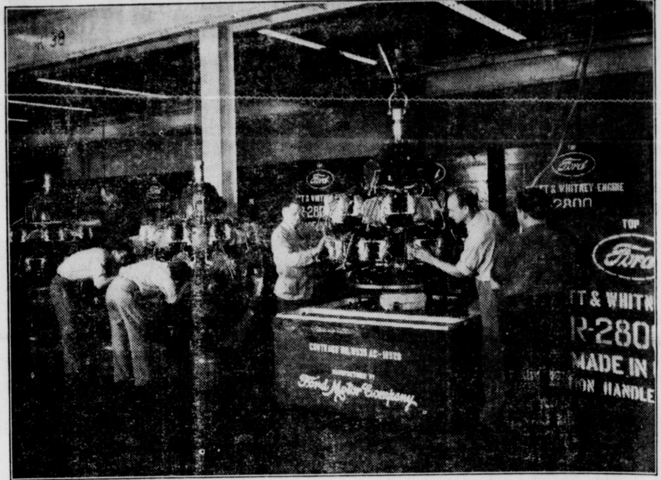
DEARBORN, Mich.—This is a corner of the Ford Motor Company's airplane engine plant, where big Ford-built Pratt & Whitney airplane engines are being packed for shipment to America's defense forces. Production has been under way for several months in this new aircraft unit of the Ford Rouge plant. Another major Ford defense project is the contract to build big four-engine Consolidated B-24 bombers. A $58,000,000 plant is under construction for this job at Willow Run, near Ypsilanti, Mich.
