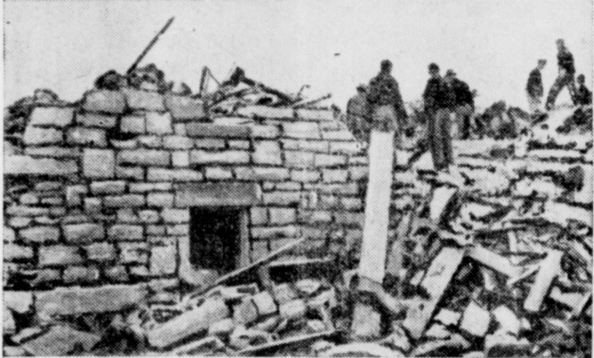
WIND RIPS ROOF FROM BARN—DEMOLISHES WAREHOUSE— Many farm buildings were unroofed or flattened by the terrific windstorm which swept central Minnesota Friday night, September 11, 1942. Scenes like this, near Maple Lake, were common. This airview shows how the wind cut across one farm, ripping off the roof of the barn and leveling the machine shed. Lower photo shows workmen starting to rebuild a wholesale firm's warehouse after a tornado struck Berryville, Arkansas. Red Cross priorities for disaster relief speeded up the rehabilitation of these communities.
