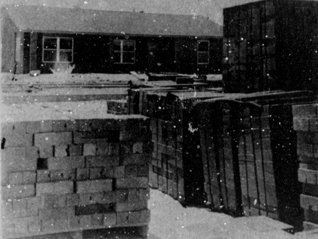
WORK AT A STANDSTILL?..... The Senior Citizens Housing project which seemed to be floundering, due to water problems received a helping hand from the Muleshoe City Council in their Tuesday meeting. (See Story P-1 for details.)
