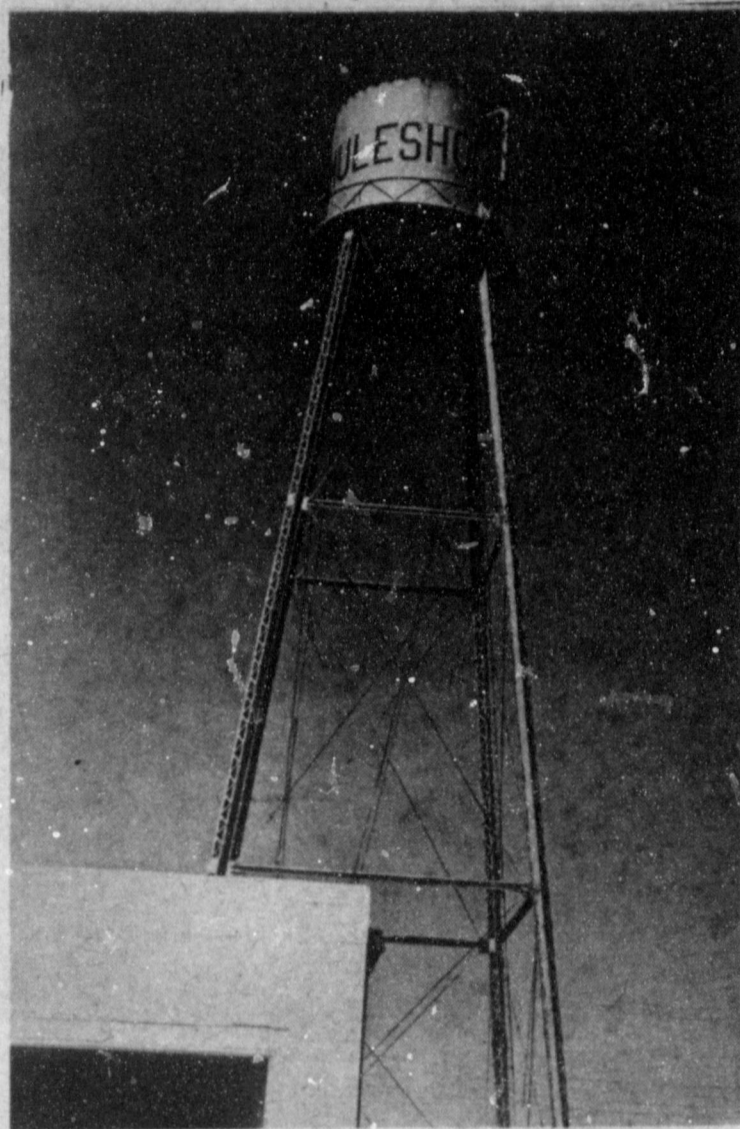
PASSING OF A LANDMARK..... The old city water tower is currently being dismantled due to the uneconomical aspects of use. The tower which is some 55 years old was in use until 1980. It was built in 1926.
