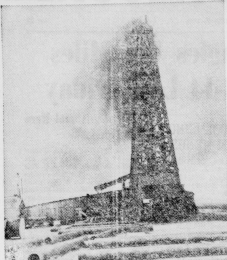
SANTA RITA, 1923 — This well drilled on University of Texas land in West Texas opened up the Big Lake field, May 28, 1923, from a depth of 3,028 feet, and drew attention to the now famous Permian Basin oil province and put the first "oil money" in the University Permanent Fund, which now holds more than $447 million from royalties, rentals and bonuses.
