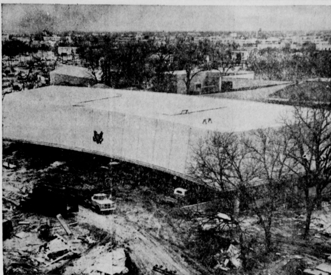
UNITED STATES PAVILION —Work on the exterior of the United States exhibit hall, one-half of a $6.75 million pavilion complex at HemisFair '68, nears completion and attention is turned to the interior design. This picture of the structure, marked by the United States Seal, was taken atop the Swiss Skyride already in operation at the San Antonio World's Fair.
