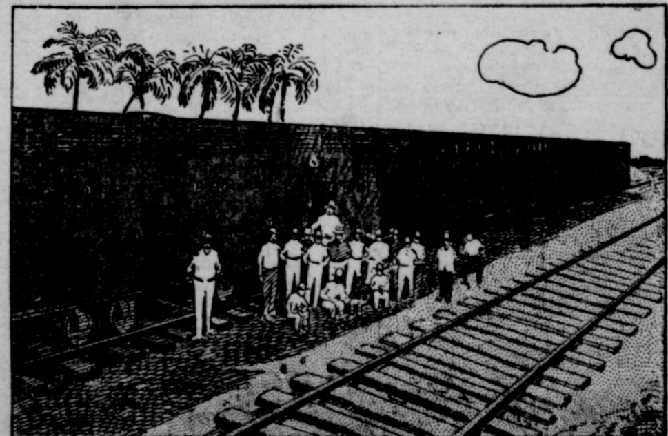
These cars are fitted up with kitchens and tables for the accommodation of the working gangs. The railroad parallels the canal and it is thus possible to place these boarding houses on wheels at the point most convenient to the laborers. The train here shown has accommodations for 40 white men and 76 blacks.
