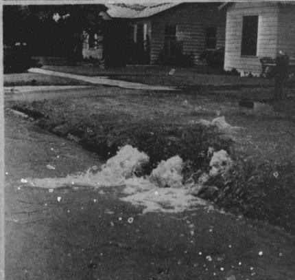
BROKEN WATER MAIN CREATES MINI-LAKE--Muleshoe Lake was nearly formed Saturday afternoon in northeast Muleshoe when a six-inch water main split open, pushing up a front yard at 118 East Cedar. Installed nearly 40 years ago, the cast iron water main finally gave in. Houses for three blocks around the broken main were without water for several hours. Around 35,000 gallons of water spurted through the main before it was all cut off and
