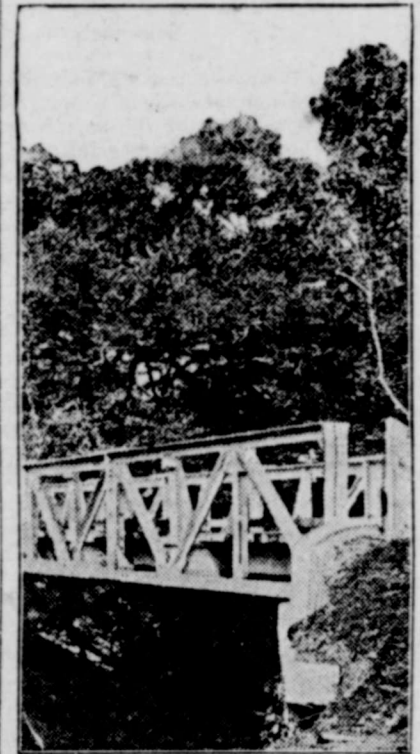
Army Sectional Bridge Erected Over Davidson River, Pisgah National Park.
