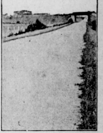
Completed Federal-Aid Road in Minnesota.
