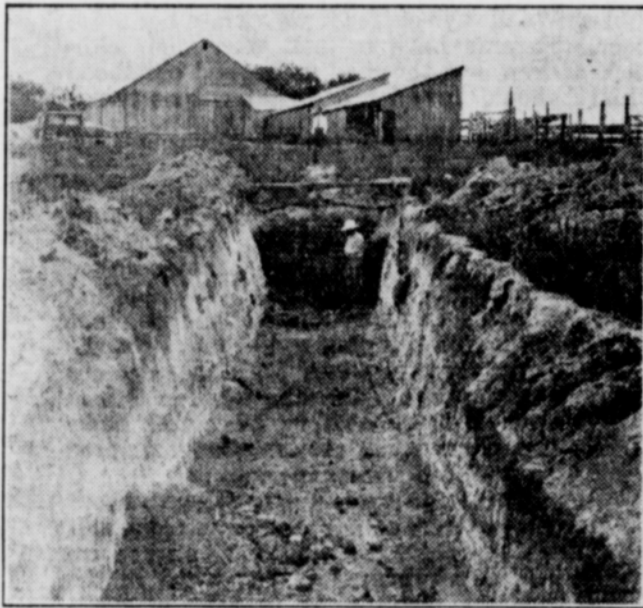
Shirley Gregg's trench silo, Gregg community, Travis county. Dug in 1935, this silo is 8 feet deep and 150 feet long. Gregg fed 300 sheep and several hundred head of other livestock from contents of the silo.
