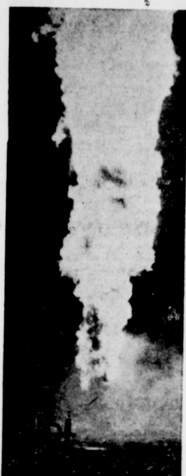
It took an all-time record blast of 155 quarts of nitroglycerin to extinguish this fire at the Continental Oil Company well at Monument Field, New Mexico. The blast raged eight days but was finally tamed by Myron M. and Floyd T. Kinley, famed fire-fighters, flown to the scene by Conoco. So intense was the heat that high-pressure fire hose carrying a full stream of water burned like paper during the conflagration.
