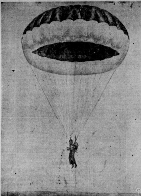
**THE LATEST IN PARACHUTES** is the Navy's new "extended skirt" type chute that will become standard equipment for pilots of jet and other high-speed planes in early 1950. The parachute, which has a 28-foot diameter, reduces the opening shock and gives a more stable descent to fliers who are forced to bail out of their fast-moving craft. (International)
