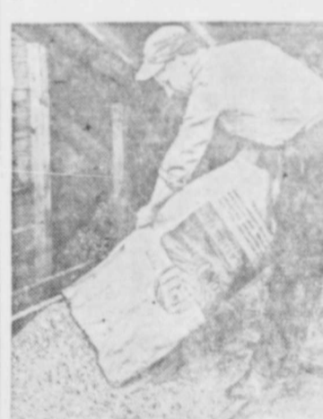
Zonolite vermiculite insulation being installed over ceiling of dairy barn at Sunnyside Farms, Oregon, Ill.
