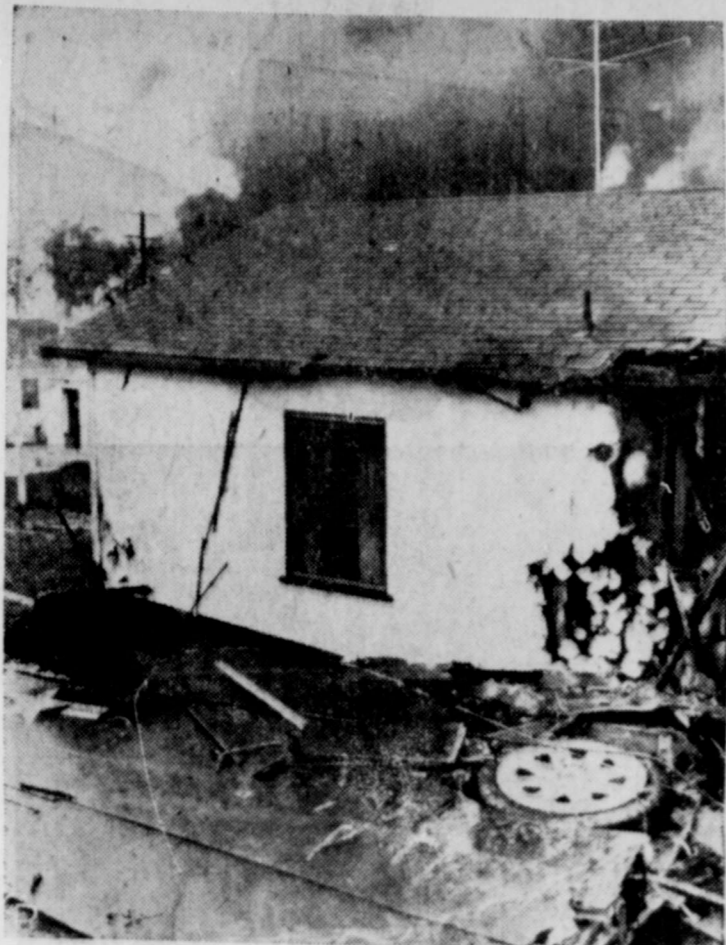
Smoke from struck oil tank rises in background, wing in foreground
