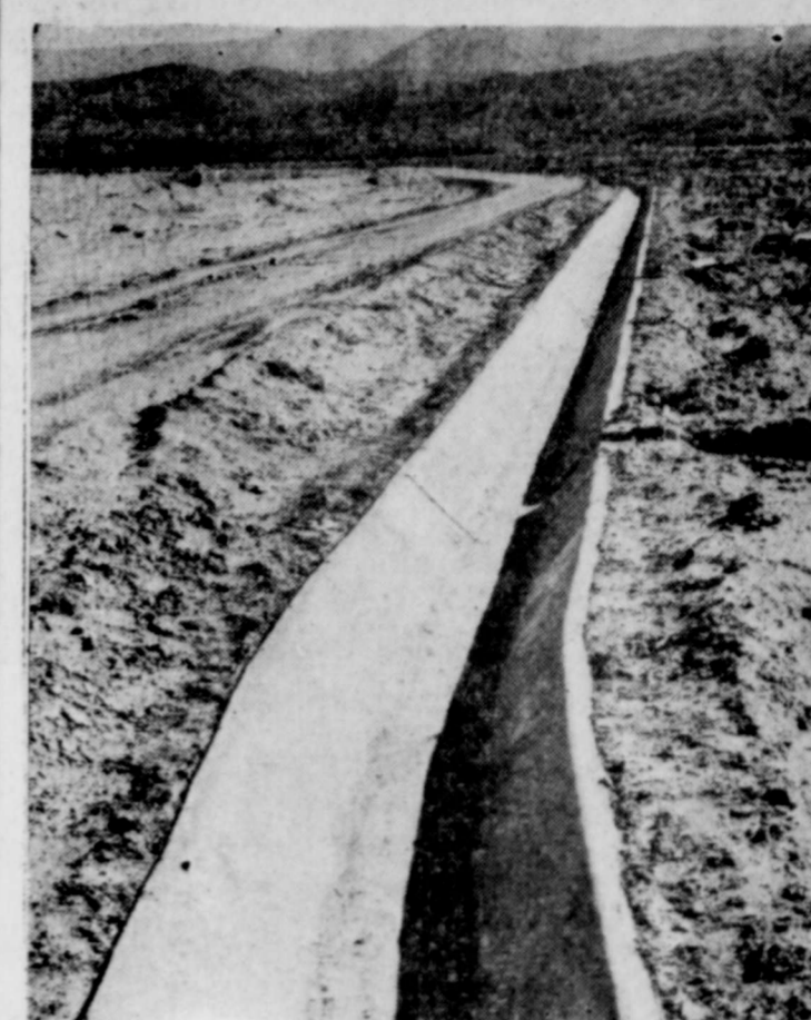
THE LINING OF irrigation ditches with concrete or other suitable materials holds water losses to a minimum, soil conservation service technicians point out. A clean, lined ditch like the one shown here, prevents seepage, reduces evaporation, and saves time and labor in irrigating.
