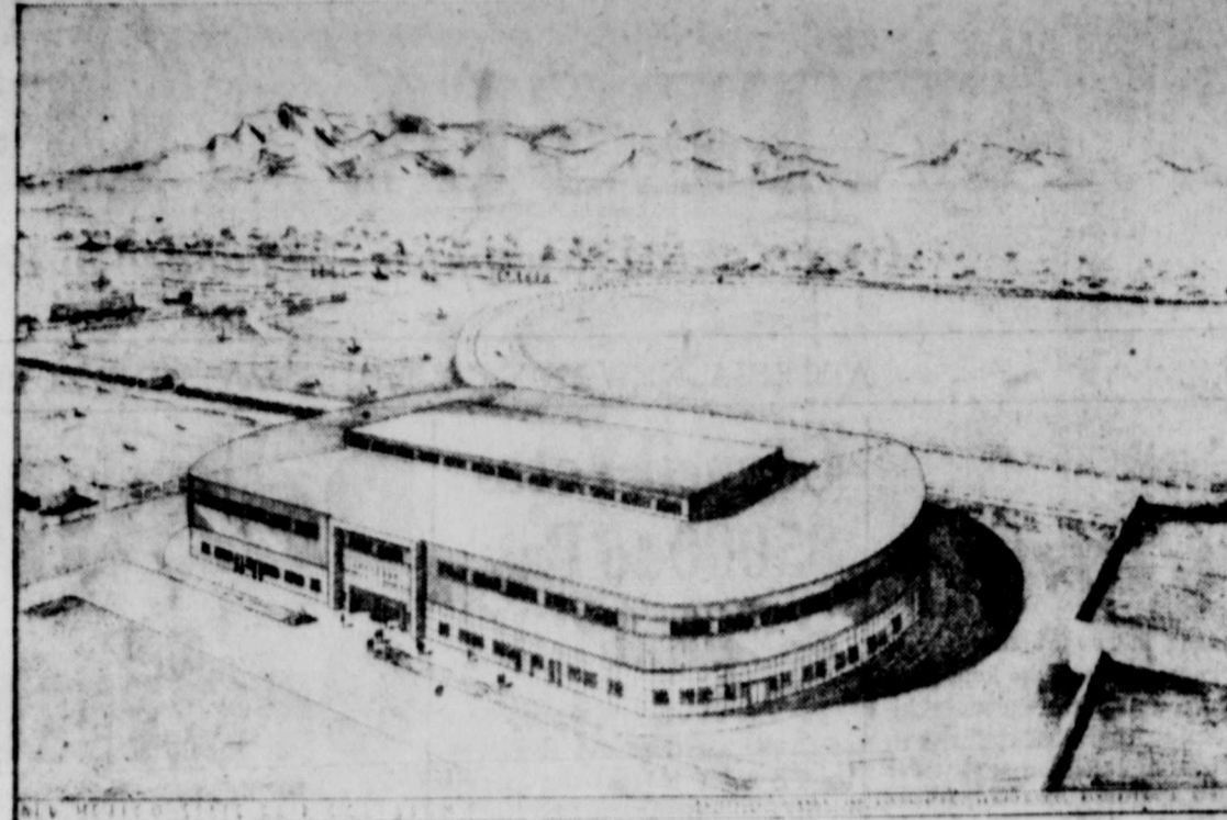
THIS is the million dollar coliseum now under construction at Albuquerque. Excavation and concrete work has been started by the Paul H. Priest firm. Many of the footings, ramps, and retaining walls will be in place by Sept. 24, New Mexico State Fair time.
