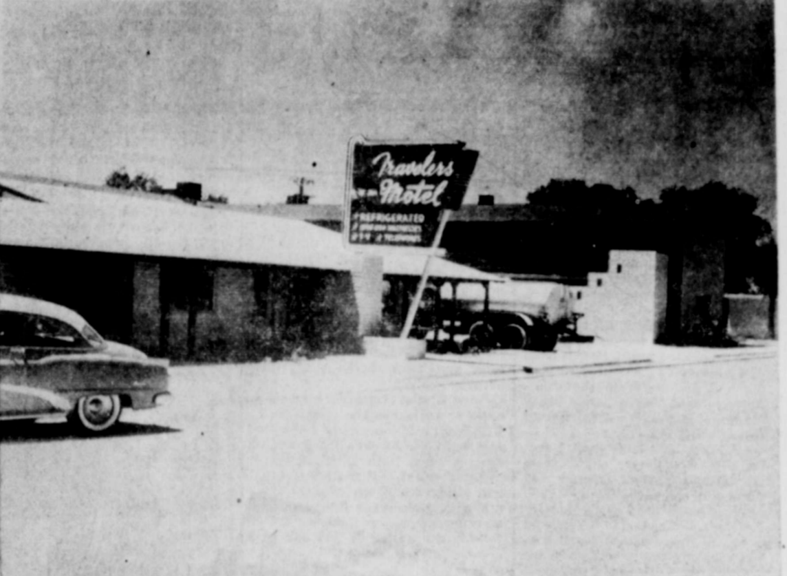
ARTESIA'S NEW Travelers Motel adds striking beauty to south highway 285. Grand opening date for public inspection is Tuesday, July 12, from 3 to 8 p. m. The Motel is located in the 900 block on South First and contains 36 beautifully furnished units with the ultimate in modern conveniences. Mr. and Mrs. Rex Holmes will conduct the initial inspection through what promises to be one of the most comfortable and beautiful motels in Artesia. The entire structure is cooled by refrigerated air conditioning. (Advocate Staff Photo)
