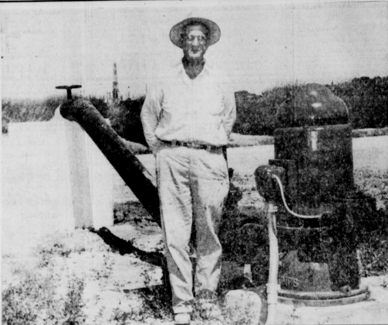
HEAVY DUTY operation is what this pump, installed by Bristow Pump Co., of Artesia is designed to do. W. M. (Bill) Jackson stands beside his new equipment now in operation on the Jackson farm southeast of Artesia. This is just one of the scores of various types pumps and pumping equipment handled and serviced by Bristow throughout southeastern New Mexico. For additional information about the pumping equipment which can best serve agricultural and industrial needs, call SH 6-2063.
