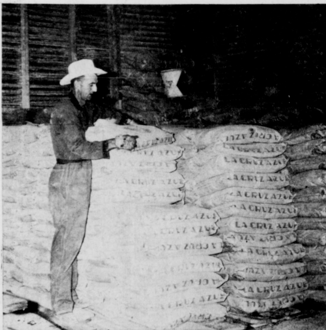
NEARLY 50 MILES of ditch liner have been laid by the Artesia firm and enormous quantities of cement have been required. Here Stiver checks over some of the cement on hand in a corner of the storage building. Purpose of the liners, all of them installed by the Fullerform method, is to increase efficiency of irrigation and prevent soil erosion. (Advocate Photo)
