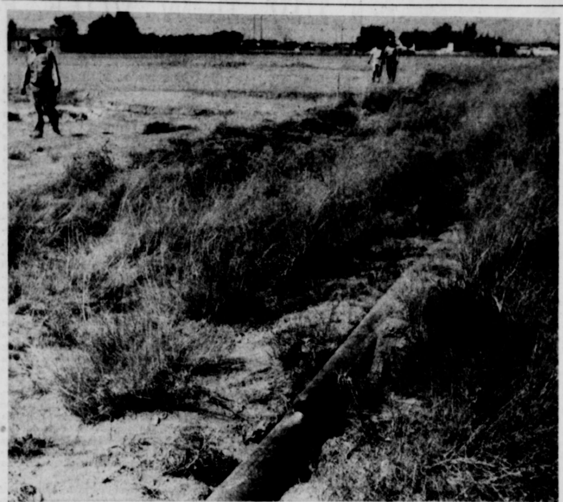
BLOWOUT —Thousands of cubic feet of natural gas are roaring out of this gaping hole in the main Southern Union Co. gas line two miles east of the city this morning. In the background, bulldozer driver Jack Privett surveys the damage done when his earthmoving equipment severed the city's main gas source. (Advocate photo)
