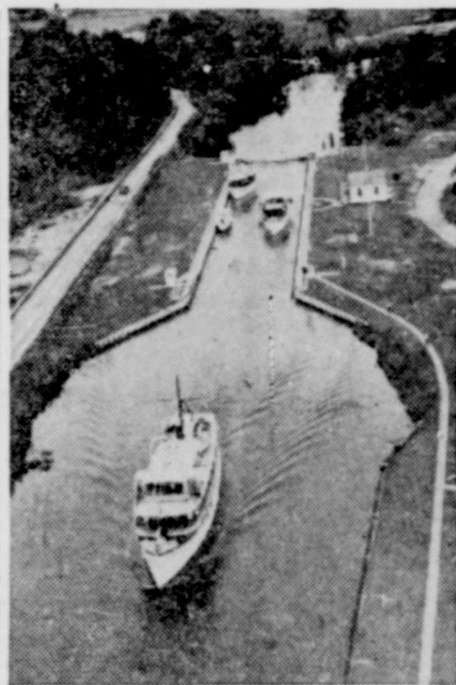
CANAL LOCKS . . . One of the two locks on Great Dismal swamp canal, which take care of a nine-foot drop in the terrain.
