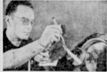
The end of a solid tube of glass is flared. This is the first step in making a tiny bubble tray used in a distillation column.
