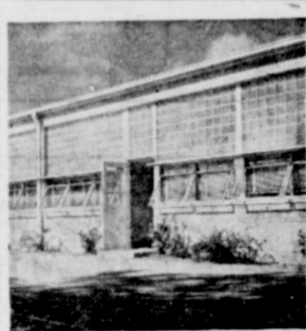
A good example of the type of building supplanting the substandard rural schoolhouse is this modern unit in Spring Branch, Comal county, Texas. All classrooms in this new school receive maximum daylight, automatically controlled to minimize glare by means of panels of light-directing glass blocks installed above clear window sash. Individual exterior doors reduce corridor traffic, offer easy access to play areas.
