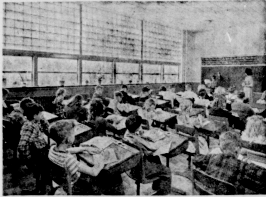
This classroom, typical of those in many new rural schools, is flooded with glareless daylight—even in remote corners. Walls and furniture are in gay pastel colors, desks are light natural wood tones, and even chalkboards are eye-comforting green instead of somber black.
