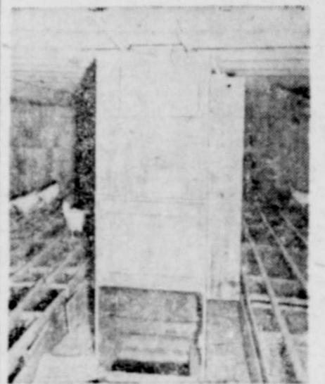
The picture above is the litter shaft invented by one poultryman. The elongated box-like structure to the right of the main structure houses the electric ventilating fan — one being located on each floor.
