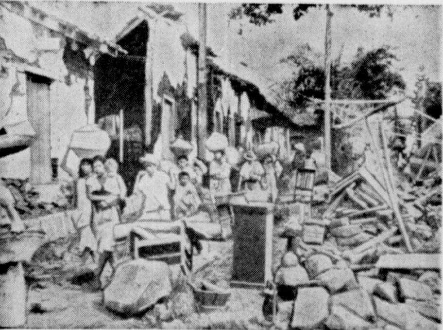
EARTHQUAKE AFTERMATH . . . Through a lane strewn with rubble, a group of inhabitants of Jucuapa, Salvador, carry whatever they can salvage as they flee to safety following violent earthquake that rocked the country recently. More damage was inflicted on the inhabitants when landslides followed the quake. The death toll was officially placed at 1,200. The Salvadoran Red Cross mobilized all its facilities to care for the injured and homeless.
