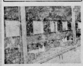
Large windows of double-pane insulating glass, admit an abundance of sunshine and daylight into the poultry house. Pictured above is the poultry house on the Henry Zumstein farm near Fairview, Ill. Agricultural engineers say this design helps to reduce moisture and sanitation problems.
