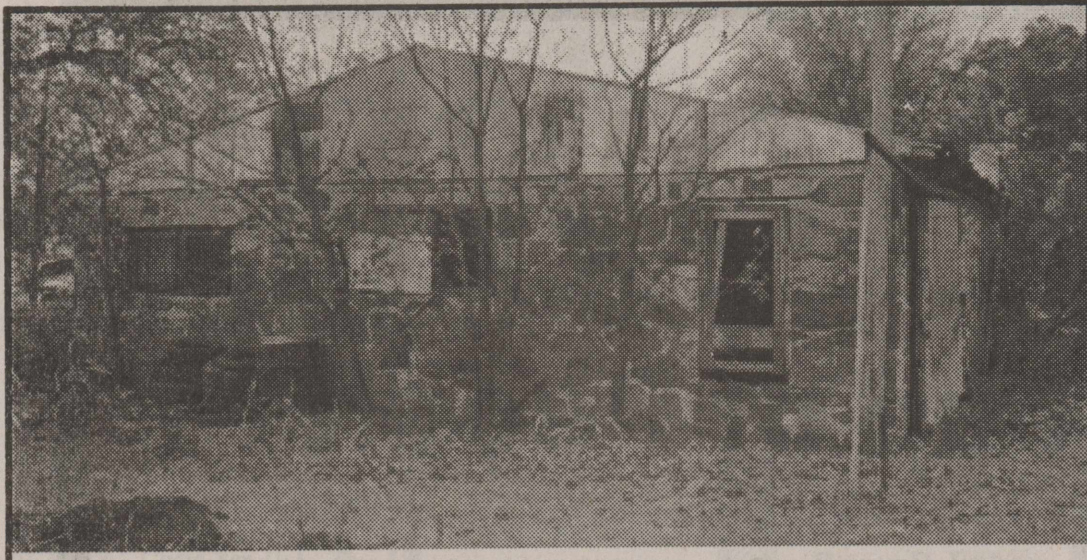
Old Building located on Hwy 36 to be Removed for the New Family Dollar Store
